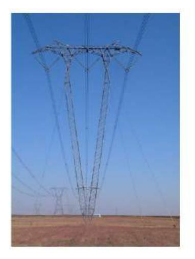
Figure A-5: Tower Type 520B (Guyed V).
