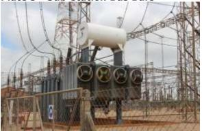
Plate 7 - Transformer showing oil reservoir and fans for cooling.
