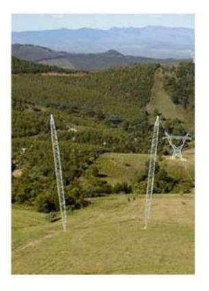
Figure A-2: Tower Type 524 (Cross Rope).
